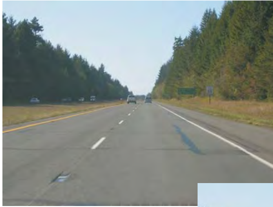
FIGURE 16 Views of North Study Corridor
