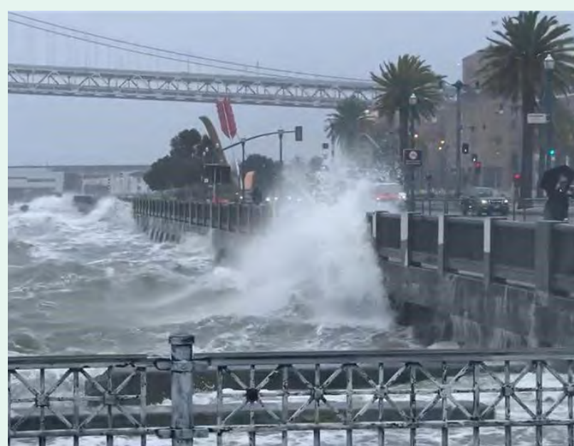
Coastal Engineering: GHD is performing an independent review of coastal hazards, SLR and tolerable wave overtopping along the Embarcadero seawall to support the Port of San Francisco Downtown Coastal Resiliency Project.
